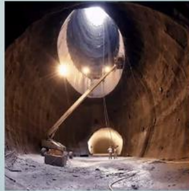
Shaft to the SSC tunnel di SSC, located at about 10 meters underground. The planned tunnel had a circumference of 87 km.
